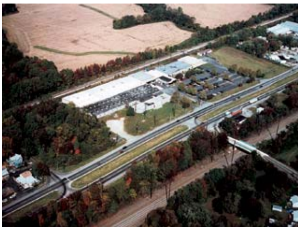
Metal Fabrication Facility
